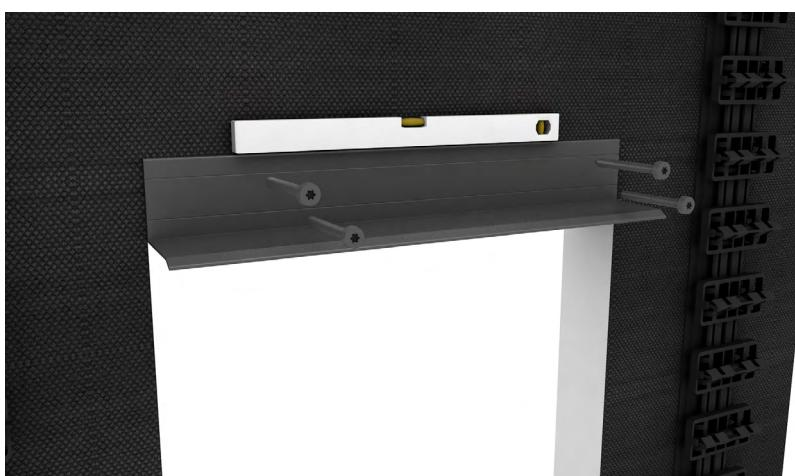
1. Position the drip edge along the façade. Make sure it is horizontal, using a level or reference surface.
